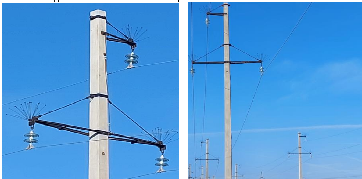
Figure 5 - Appearance of constructed power transmission lines with ASHT wire.
